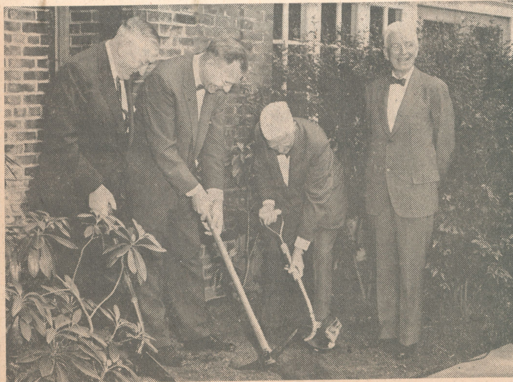
Here is the actual ground breaking for the new Wilkes College Science Hall. Scene was in rear of the Butler and Ashley build-
