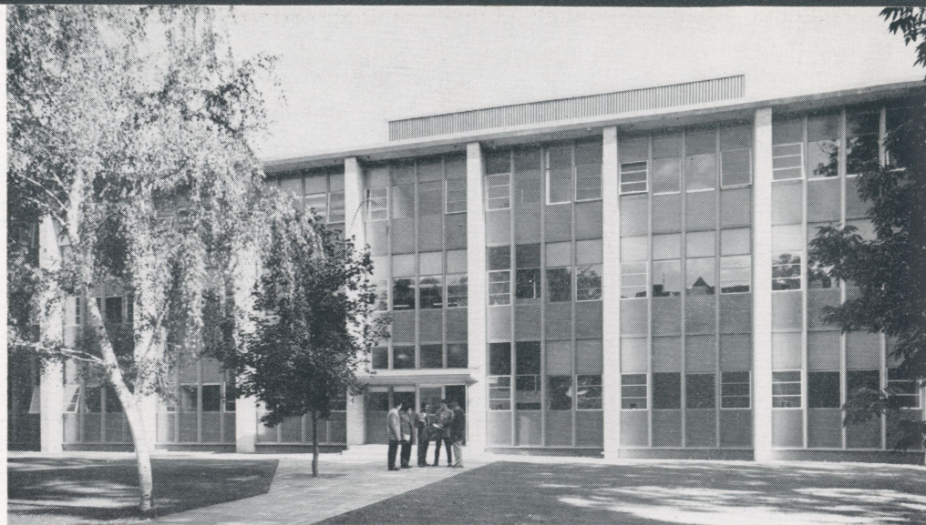
● A frontal view of Stark Hall. Though limited by its setting and surrounding undisturbed trees, this view shows well its basic design and construction. The three-story and basement building is 60' x 210' and encompasses some 56,460 sq. ft. Of reinforced concrete construction, white Colonial brick piers set off the enameled steel supports and porcelain steel panels with alternating bands of clear glass and blue textured heat-absorbing glass.
