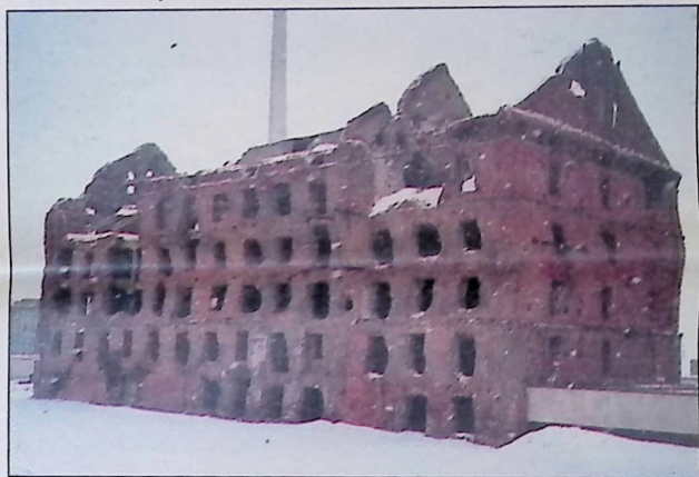
Bombed-out building left standing as a stark reminder of the Battle of Stalingrad.
