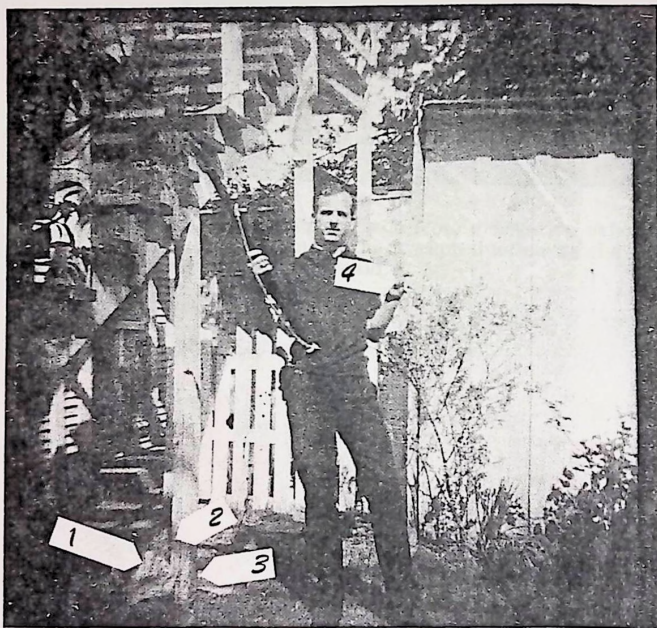
FIGURE RIT 5-1A.—Print made from the negative of Oswald (CE-749) for scratch comparison with a negative exposed in the Oswald camera at RIT. Four prominent scratches were found to be in the same locations on both prints.
