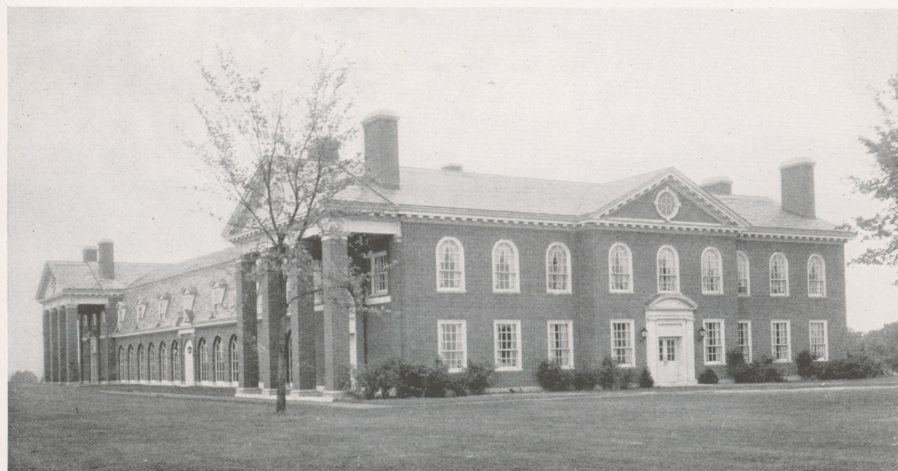
THE CHARLES P. VAUGHAN LITERATURE BUILDING
