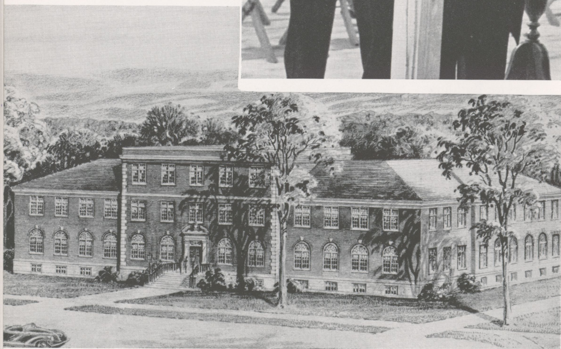
A dynamite charge sends up the earth as ground is broken for the new Engineering Building. President Marts watches as Dr. Charles A. Lindemann sets off the blast. The Engineering Building as it will look when completed.
