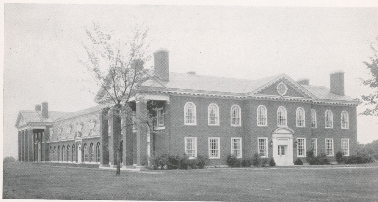
THE CHARLES P. VAUGHAN LITERATURE BUILDING
