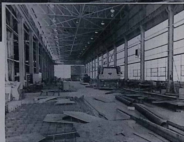
Shown here in two October photographs is an over-all view of Dor-Oliver's Hazleton, Pa. Plant and an interior of a portion of the new Structural
