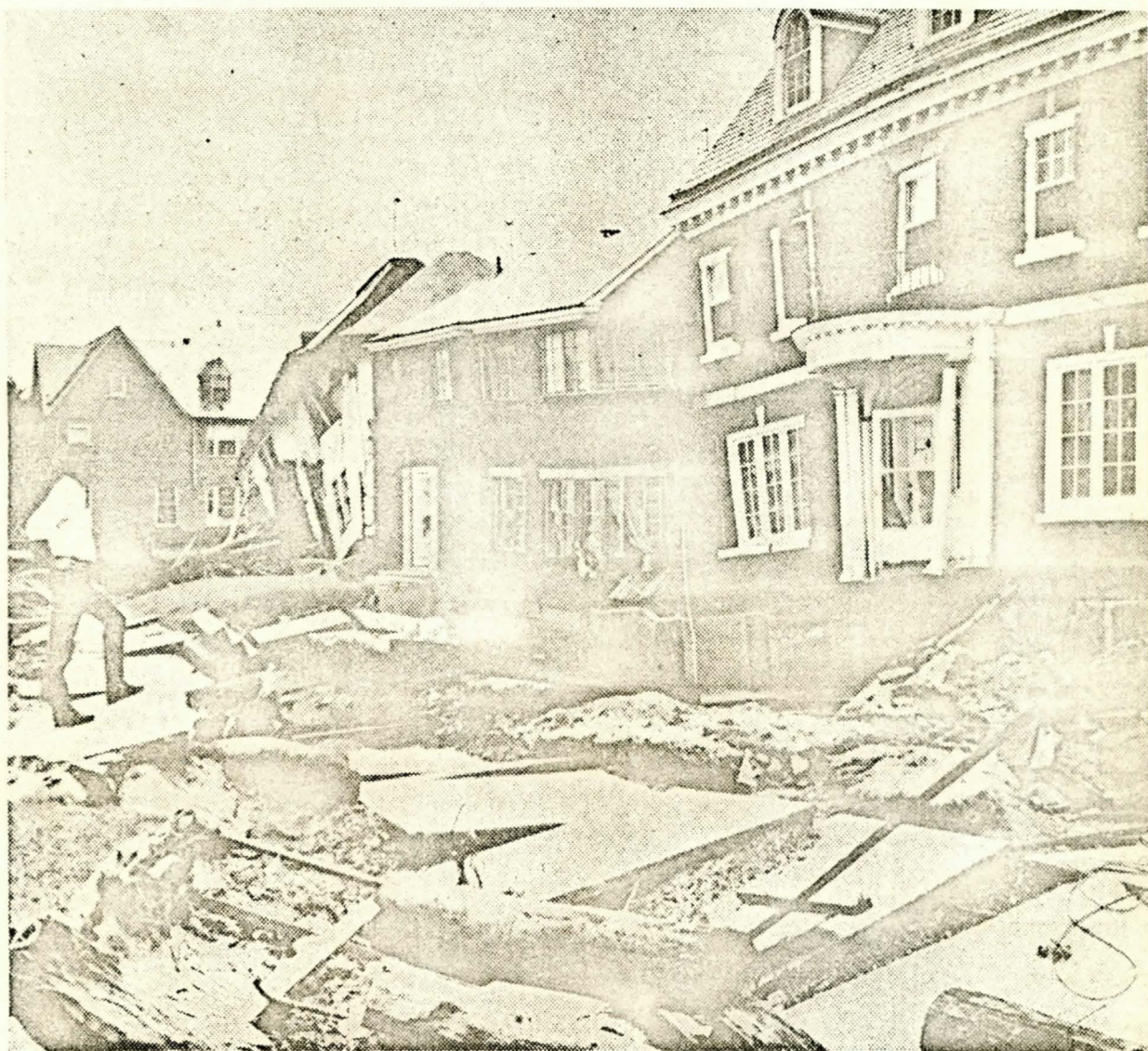
Homes in Wilkes-Barre, Pa., stand precariously, their foundations damaged by flood. Debris covers the street.
