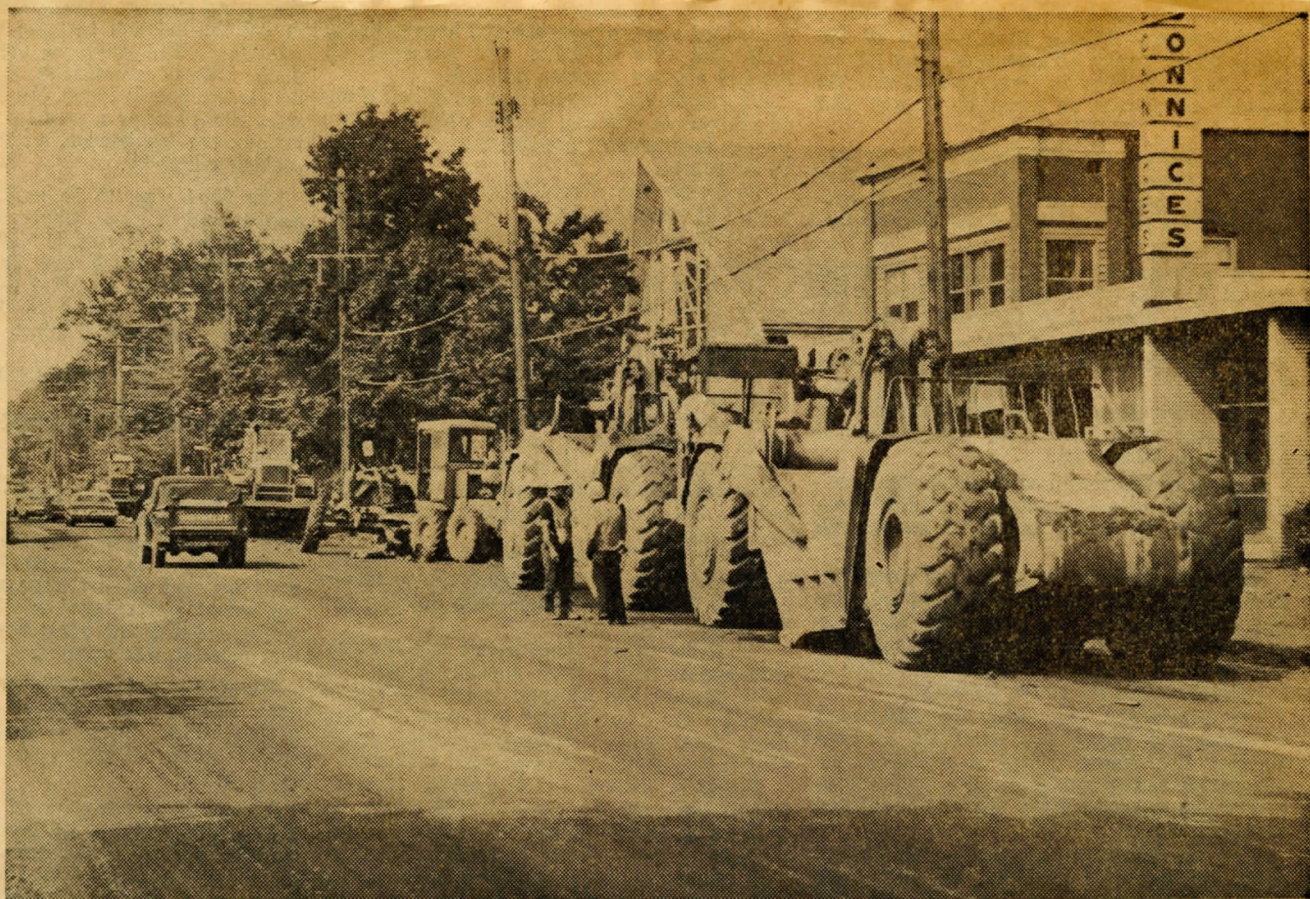
EARTHMOVERS USED — These large earthmovers, shown here on Wyoming Avenue in Forty Fort, were among the pieces of heavy equipment pressed into service to clean mud and debris on the West Side.
