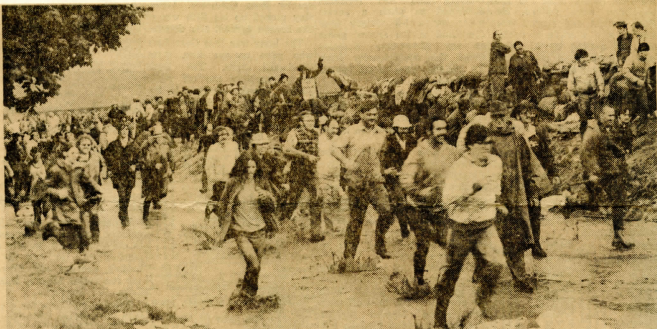
The River won. The dike has been breached and volunteer sandbaggers in the area run for safety after orders were given to evacuate the area. The evacuation sirens were sounded at 11:14 a. m. These pictures were taken by Jack Walton of Wilkes-Barre, Associated Press employee, and were widely used in Saturday and Sunday editions of the AP.
