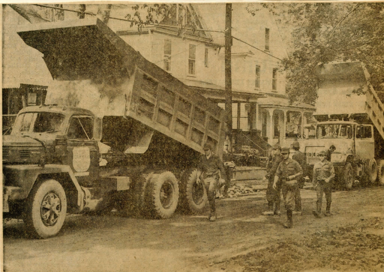
FORTY FORT CLEANUP — National Guardsmen from the western part of the State are shown loading debris
