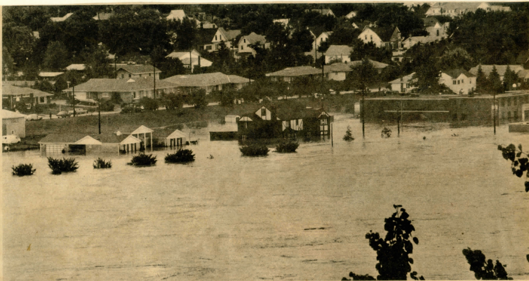
View of West Pittston from Pittston Hospital
