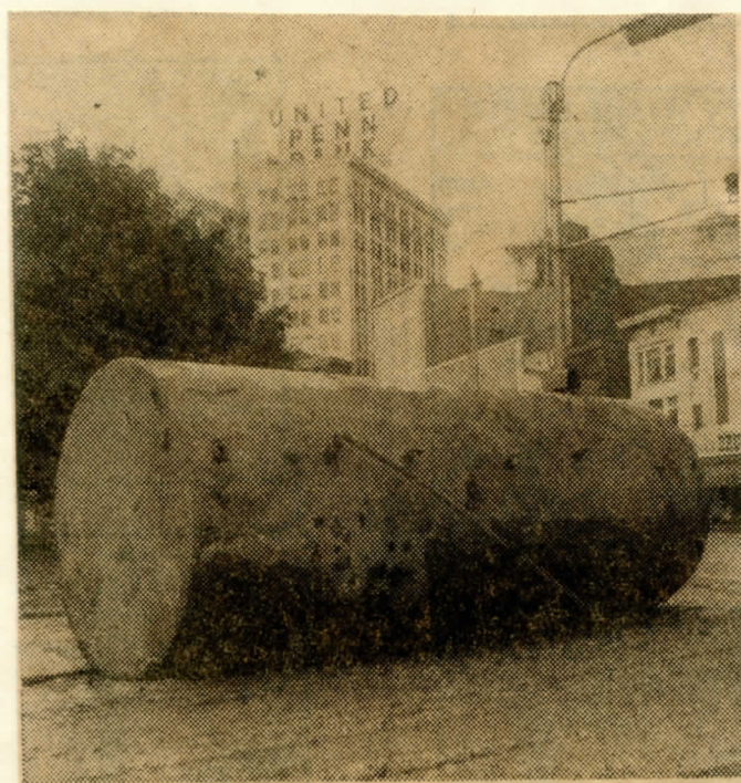
ORIGIN UNKNOWN —A 20,000-gallon service station gasoline tank, lost but not unnoticed, sits in the middle of Wilkes-Barre's Public Square. Military police said the tank will be moved today.
