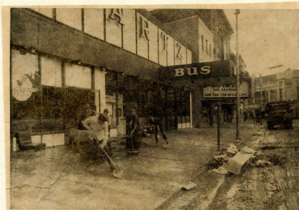
WASTING NO TIME —Employees of the Central Travel and Ticket Agency in the Martz Building on Public Square, Wilkes-Barre, push mud and debris from the building and air soggy furniture.
