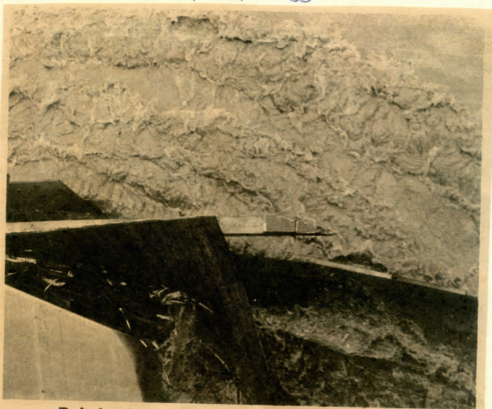
Debris slams pier of Fort Jenkins Bridge
