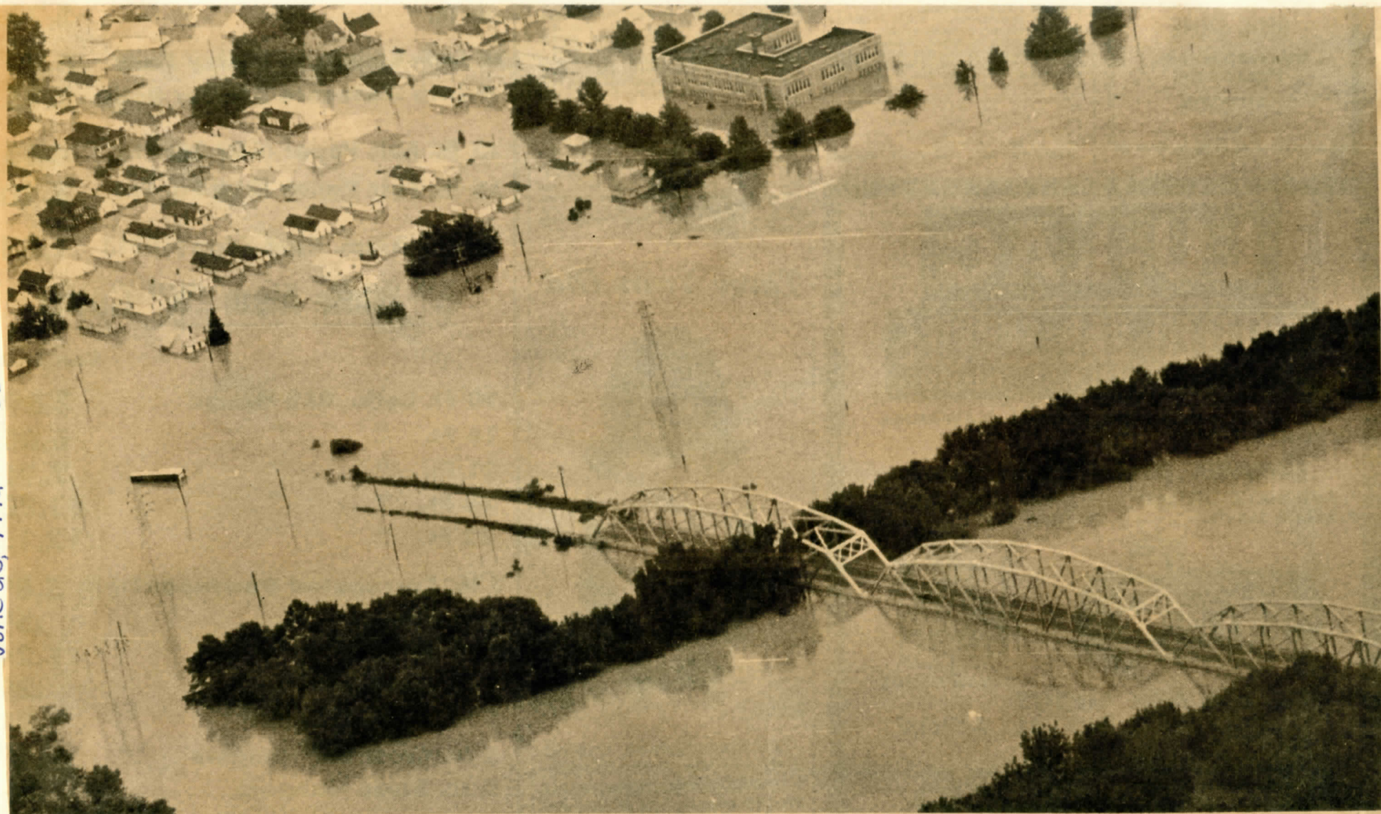
Carey Avenue Bridge, Wilkes-Barre
