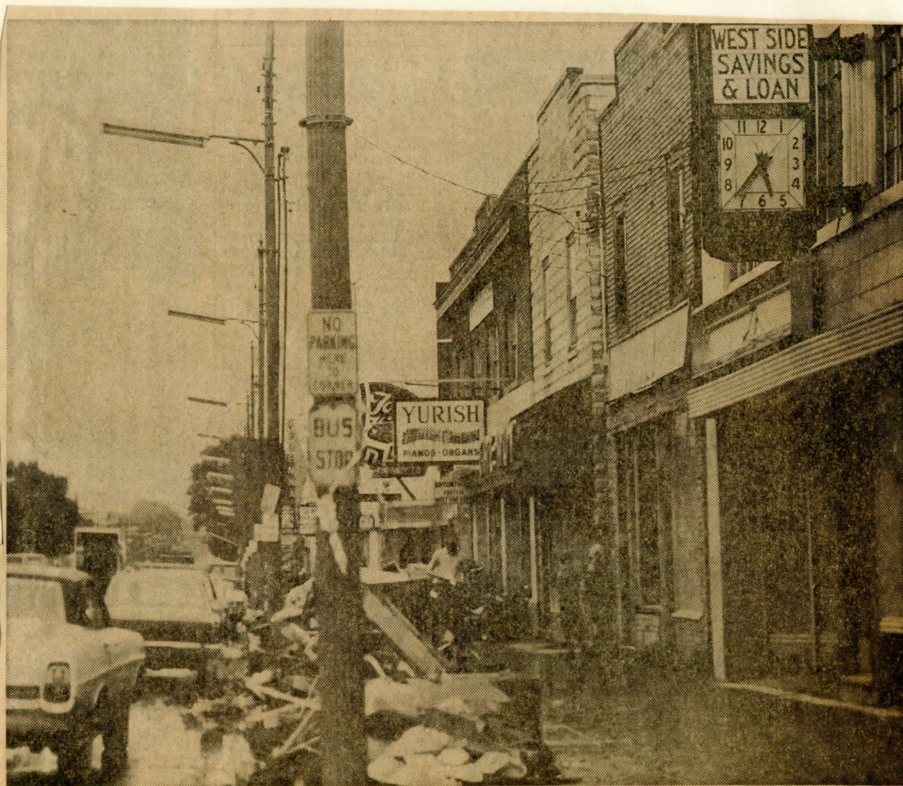
KINGSTON CORNERS . . . Debris littered the curbline at Kingston Corners in the wake of the flood. This picture was
