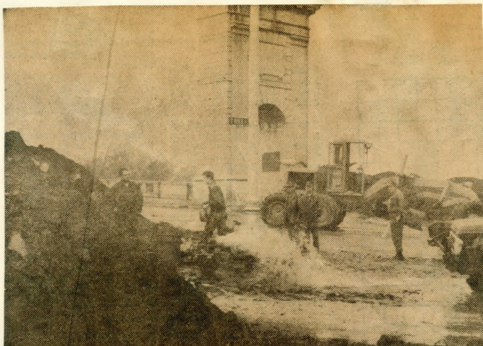
VITAL BRIDGE OPENED —Workmen pump water from the dike area on S. River Street at the eastern end of the Market Street Bridge to Kingston. Watching the clearance operation are Joe Juliano, John Migliore and William Kelly from the Seabee unit at the Naval Reserve Center, Avoca.
