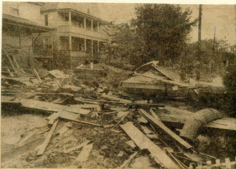
KINGSTON STREET SCENE —Entire porches, roofs, furniture and other debris blocked Goodwin Street in Kingston Monday, one block off E. Market Street. Only the chirping of birds broke an eerie silence.
