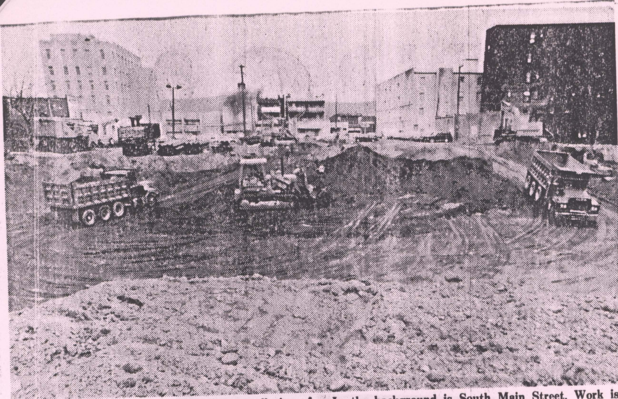
EARTH MOVING — Pictured is the overall view of the space that the new Wilkes College gym will occupy. In the background is South Main Street. Work is scheduled to be completed by the end of 1988 or 1989.
