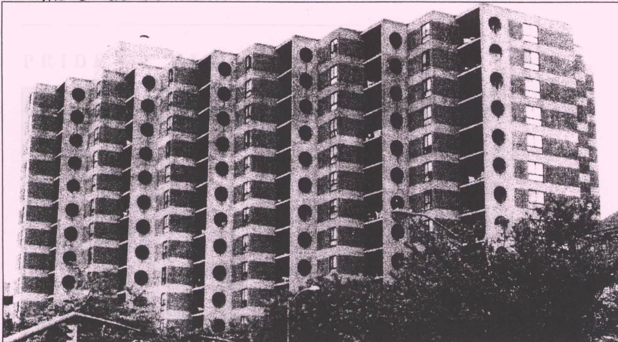
Ten East South Street Apartments
