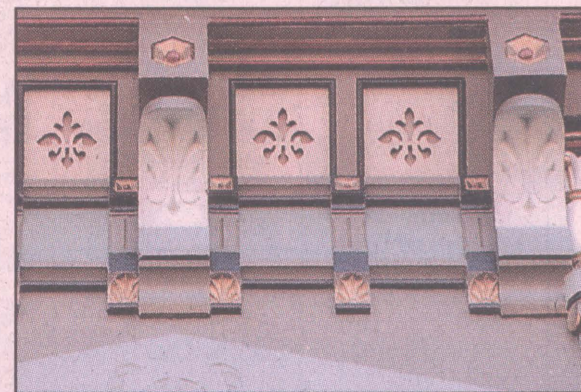
Intricate moldings surrounding the outside of the building have been carefully painted in a trio of colors to blend with the rest of the building.
