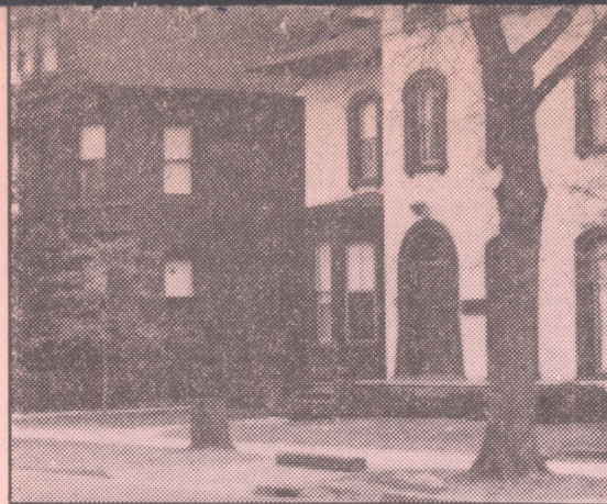
Old college buildings that were demolished for learning center
