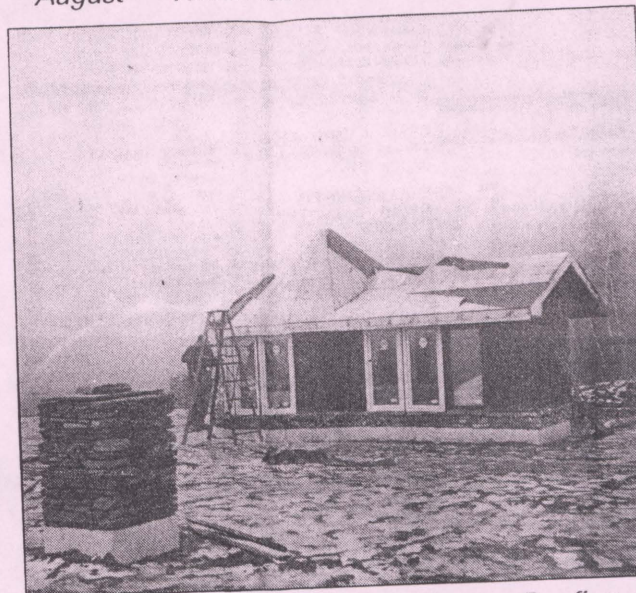
December — Entrance Gets Copper Roofing
