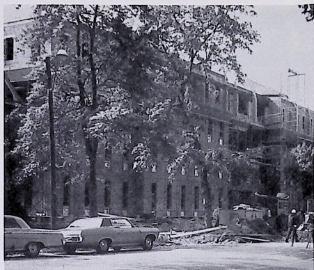
LEARNING CENTER COMPLEX (currently under construction)
