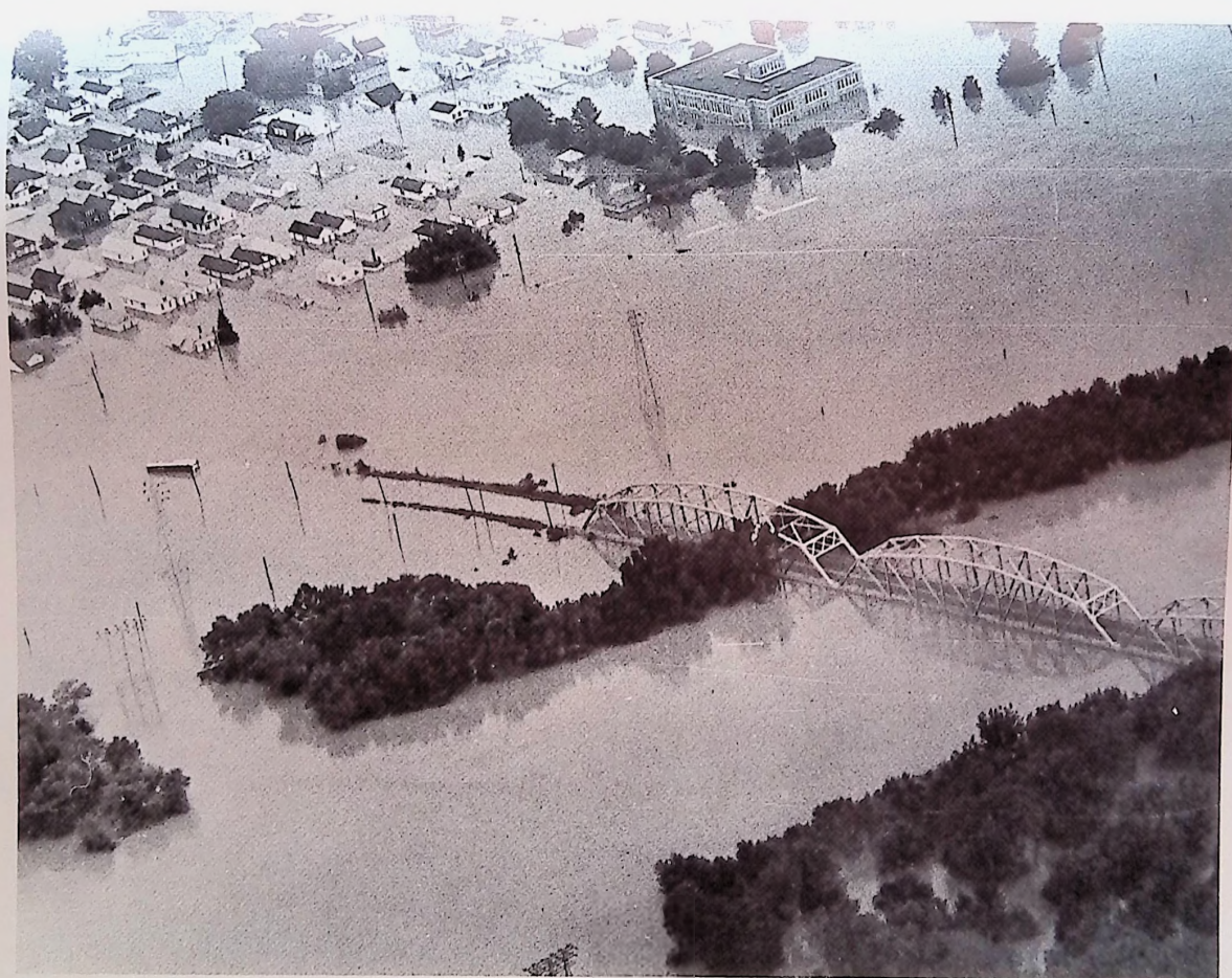
Carey Avenue Bridge
