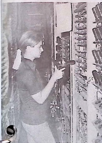
Hairdryer used on Bell wiring.
