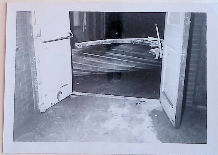
Photo # 3, 4 – View from doorway of warped flooring only contained by steel building frame. Cross angled layered sub-floor waves!
