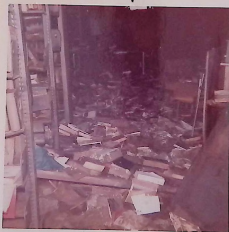
Photo # 6, – Mud and flood debris after water receded.
