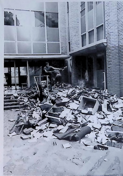
STARK HALL LOADING DOCK AND CHASE HALL WORKERS
