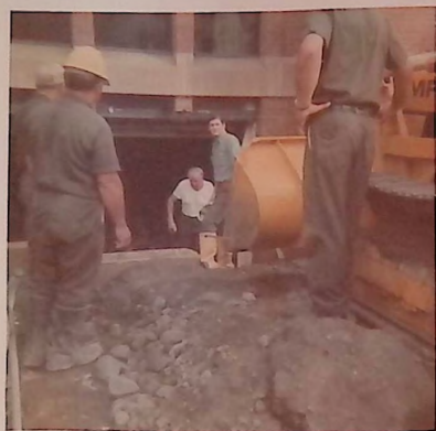
Photo # 7, 8, 9 - Entry created through basement wall from street for Payloader entry to remove debris.
