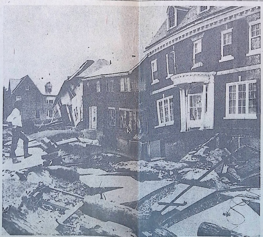
Homes in Wilkes-Barre, Pa., stand precariously, their foundations damaged by flood. Debris covers the streets.
