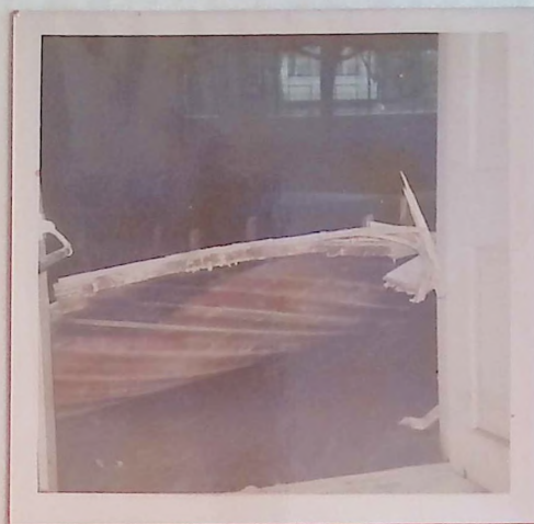
Photo # 3, 4 – View from doorway of warped flooring only contained by steel building frame. Cross angled layered sub-floor waves!
