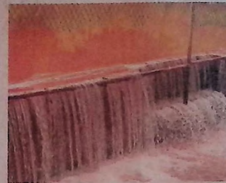
Acid mine drainage flows through the Askam Oxidation treatment center on Nanticoke Creek.
