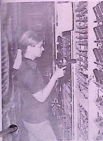
Hairdryer used on Bell wiring.
