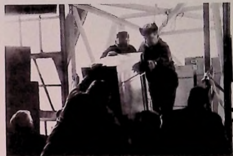
• Equipment goes up window ramp onto a waiting "Crane Cage."
