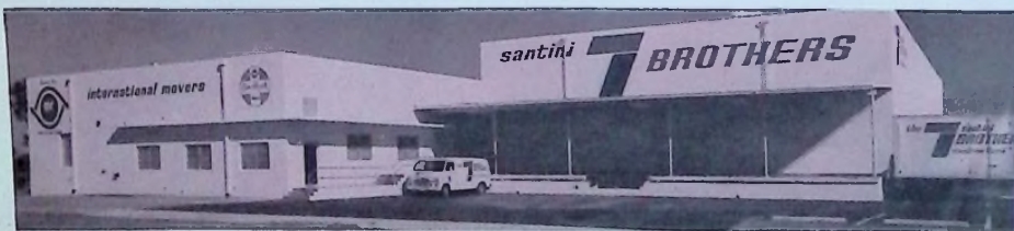
• Full front view of new West Palm Beach terminal.
