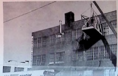
• "Crane Cage" is perched outside building to lower heavy equipment down the side of building and into waiting van.
