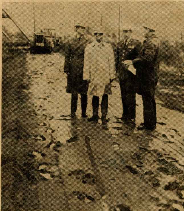
INSPECTION OF DIKE —Frank Carlucci, personal representative of President Nixon, inspects a section of the Susquehanna River dike between the Carey Avenue Bridge and Breslau Bridge which has been raised two and one-half feet.
