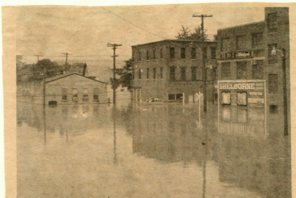
Shelbourne Corp. with water covering first floor on Penn Ave., Wilkes-Barre.
