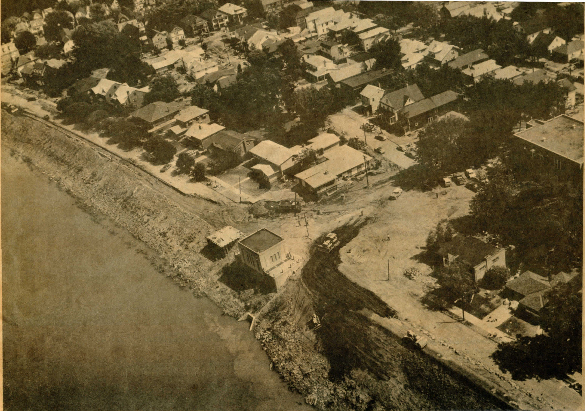
Aerial view of corner of Old River Road and Riverside Drive in South Wilkes-Barre near the pumping station. Picture shows progress as engineers work to repair the dike where river burst through.
