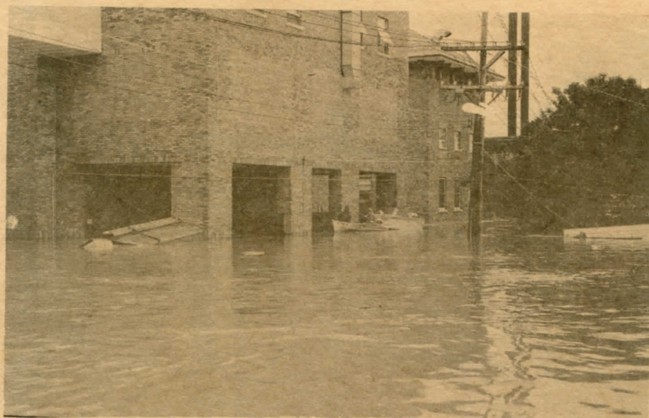
Rear of Nesbitt Hospital as flood waters reach high mark.
