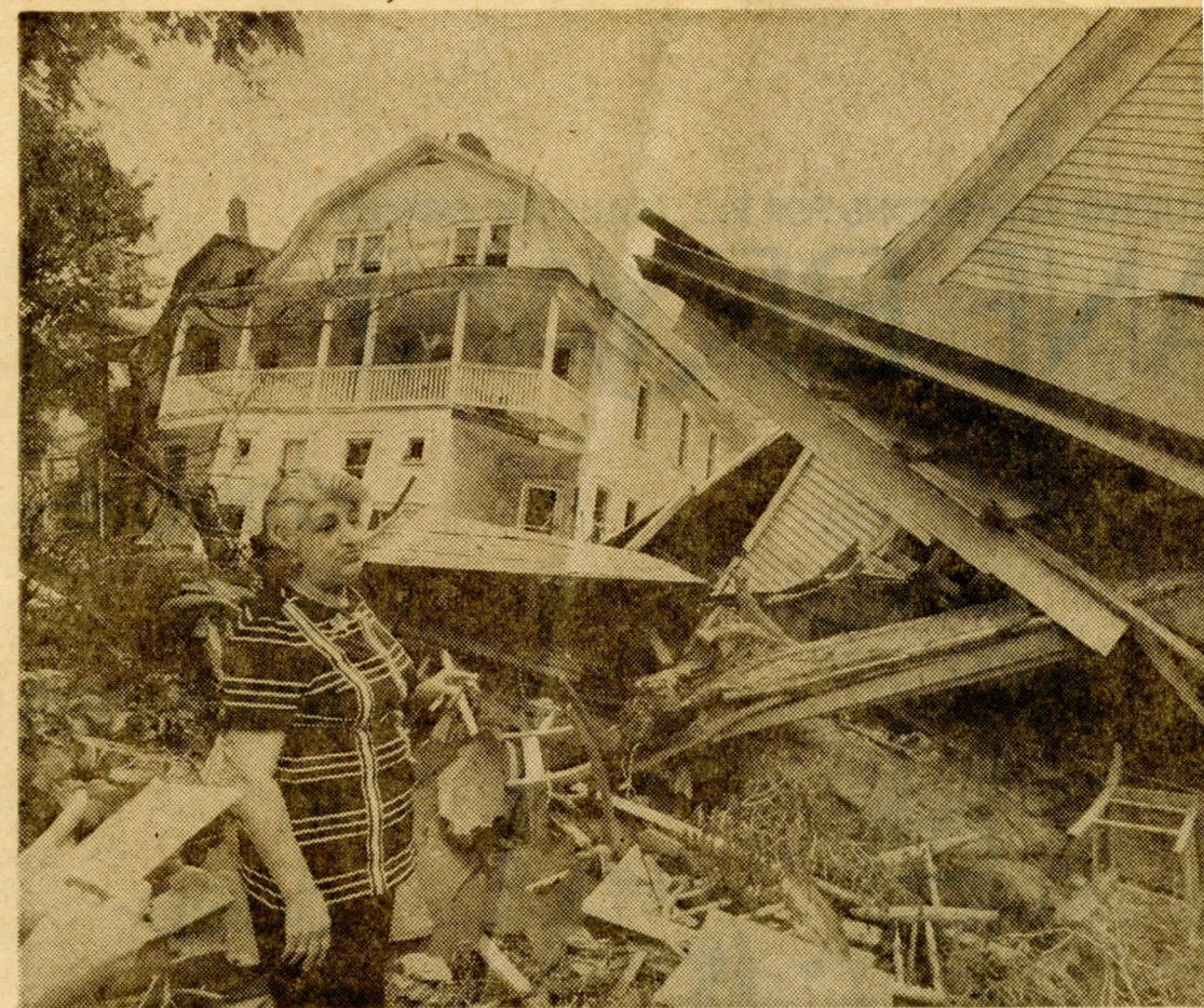
Mrs. Ann Ank in front of some of the damaged houses in Wilkes-Barre, Pa., that have not yet
