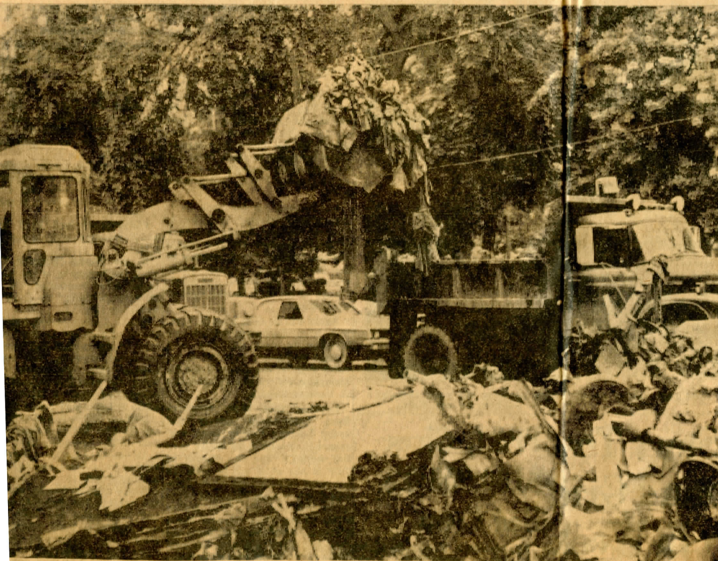
MECHANIZED EFFORTS — Heavy machinery was employed today to begin clearing rubble discarded on Public Square, City.
