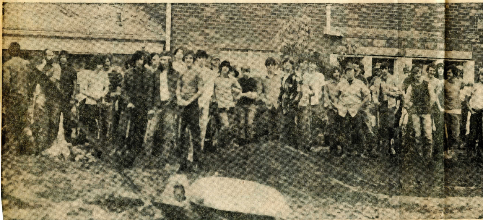
VOLUNTEERS REST —Volunteers in the clean-up effort in Gateway Apartments take a cleaning mud from roadways break from the massive job of in the Edwardsville complex.
