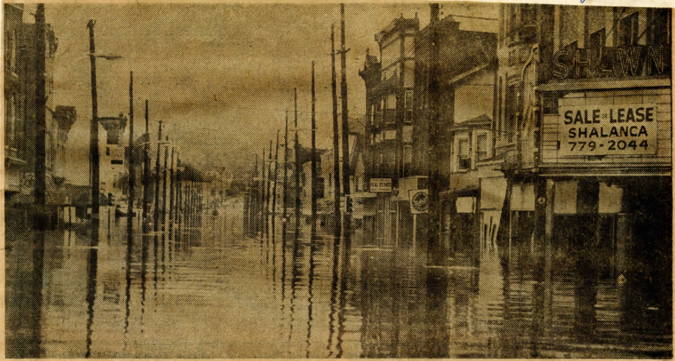
Main Street, Plymouth inundated by flood waters.
