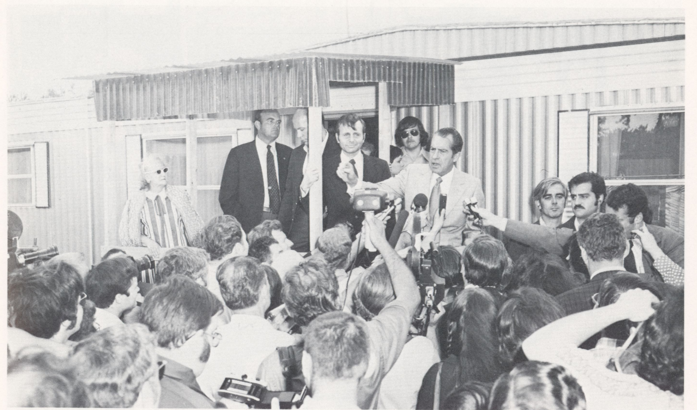
At Mobile Home site
