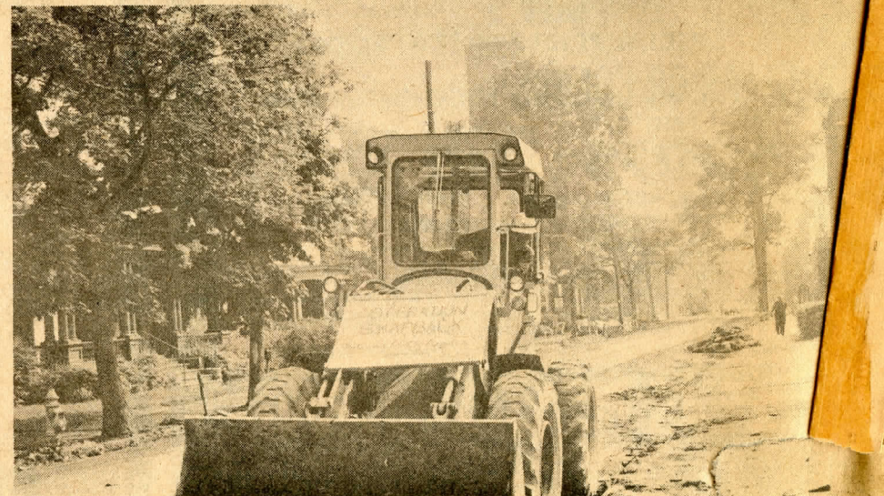
This front end pay loader immediately got into the spirit of "Operation Snapback." It is driven by Fred Sislo, Moosic, who is with the Pennsylvania Department of Highways out of Clarks Summit.
