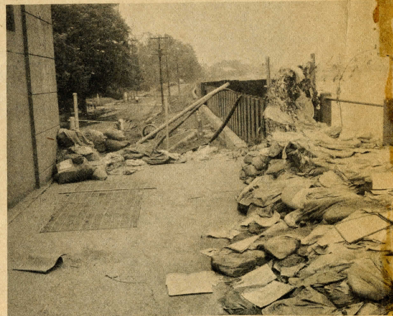
At pumping station, near Ross Street, remains of sandbags and other materials used in futile attempt to stem overflow of river. Note the height of the green metal dike, which is a couple of feet higher than the level of the pumping house where flood waters came rolling in. The metal dike was erected so that if subsidence took place the level of protection would remain at regular dike level. Hoses were used to pump river back over dike into the flowing stream.
