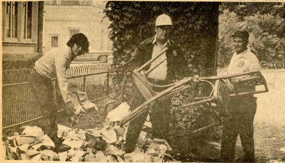
Part of the rubble is being stacked, sorted and sometimes discarded by, left to right, Rob Jemio, a senior from Bolivia; Nelson Carle, Wilkes superintendent of buildings and grounds; and John Yanchick, Swoyersville, a member of the college crew, who refused to quit "Operation Snapback" despite an injury which left him with his right arm in a sling.
