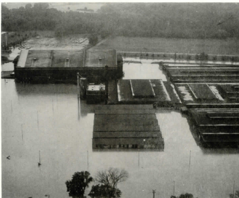
AIR NATIONAL GUARD FACILITIES AT THE HARRISBURG INTERNATIONAL AIRPORT, MIDDLETOWN WERE HEAVILY DAMAGED BY FLOOD WATERS.
