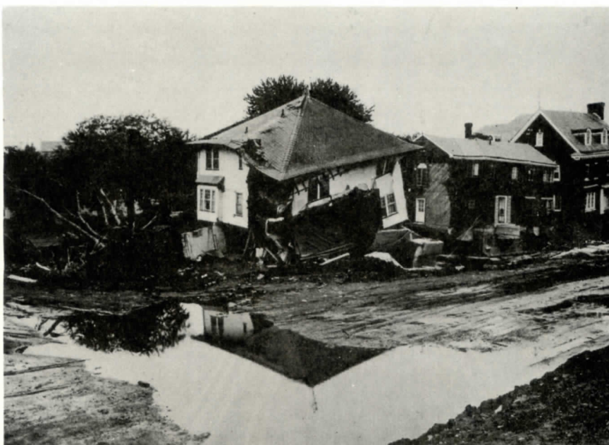
WILKES-BARRE...DESTRUCTION CAUSED BY ONRUSHING WATERS OF THE SUSQUEHANNA RIVER WHEN THE DIKE BROKE IN THE SOUTHERN PART OF THE CITY.
