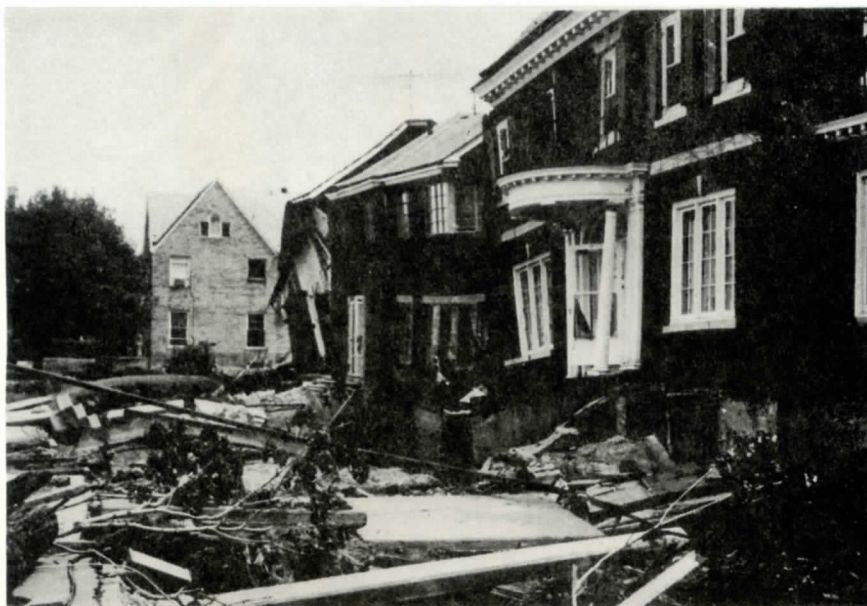
WILKES-BARRE...A RESIDENTIAL AREA TURNED TO RUBBLE.
