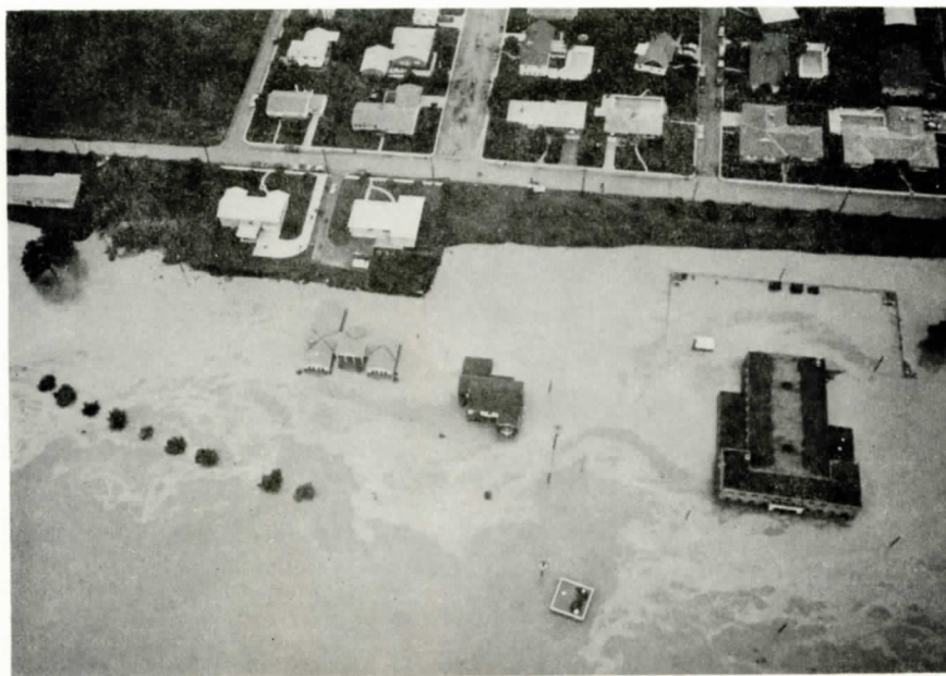
WEST PITTSTON...ARMY NATIONAL GUARD ARMORY SHOWN AT LOWER RIGHT OF PHOTO HAD FIVE FEET OF WATER ON FIRST FLOOR.
