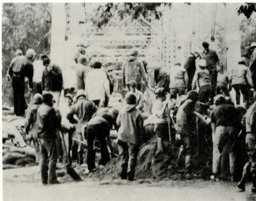
WILLIAMSPORT...THE FILLING OF SAND BAGS TO REINFORCE DIKES WAS TRIED IN THE EARLY STAGES.
